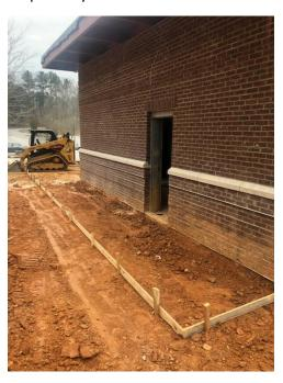
Figure 1 S. Atl –Grading for Sidewalks
